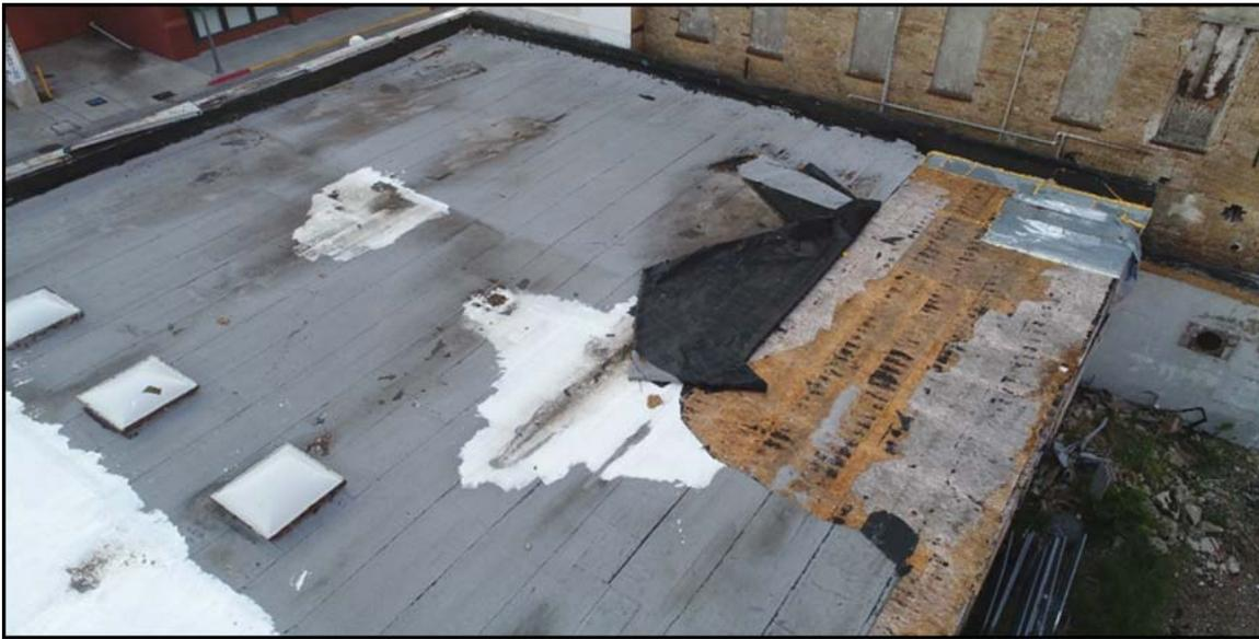
Roof deemed unsafe to inspect. A drone was the best and most timely way to inspect the damage.
