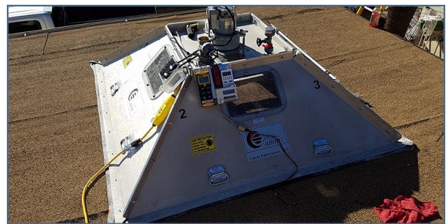
Figure 6 - Vacuum uplift testing.
