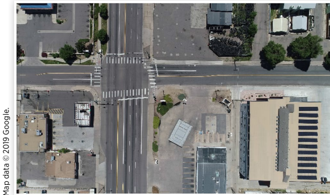
FIGURE 4 Intersection of Federal Boulevard and West Kentucky Avenue.
