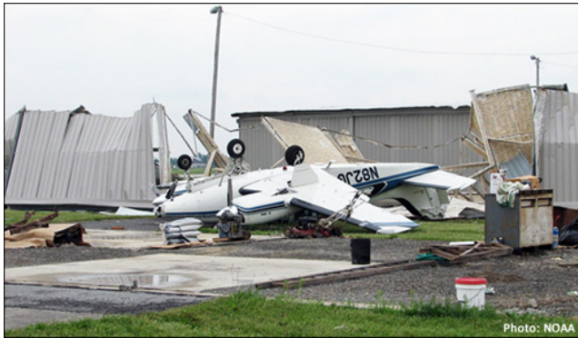
Figure 4 - Wind damage (Photo: https://www.weather.gov/safety/wind ).
