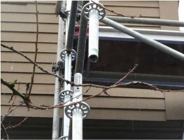
Figure 5 - Decoupled verticals due to omission of locking pin.
