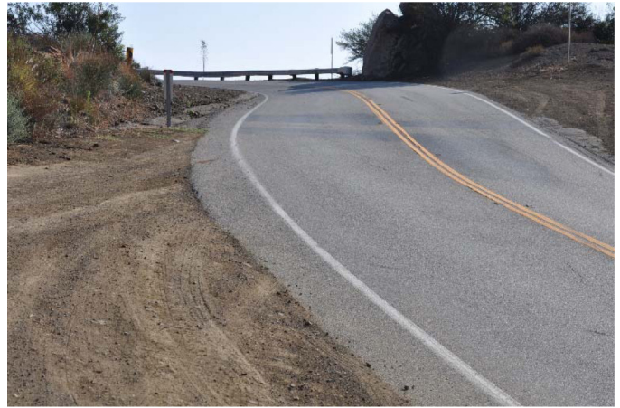
Figure 3. Inspection Photograph of the Ascent into Edwards Corner
