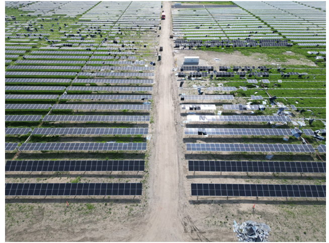
Figure 2 - High wind damage to a solar panel farm.
